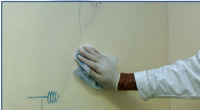
Graffiti removal in progress
